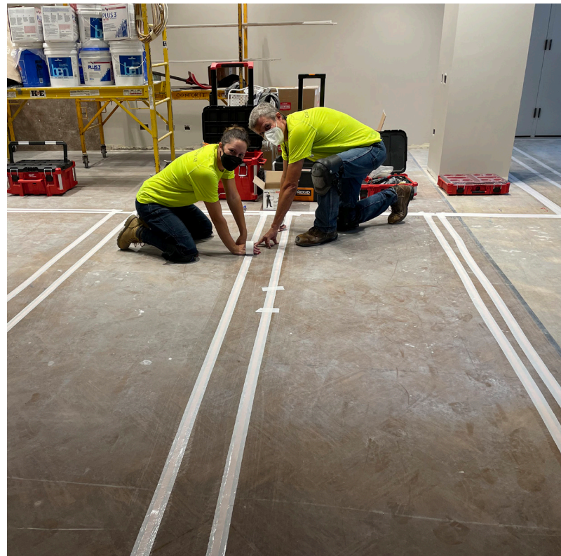
▼ Installing the hearing loops system
